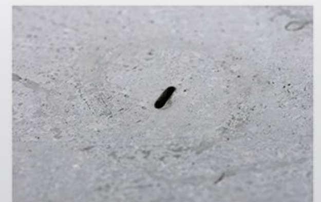
Low pressure piercing - ON
